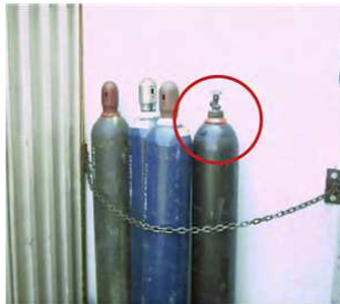
Safety cap missing
