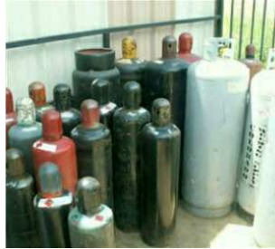
Cylinders not secured to prevent tipping
